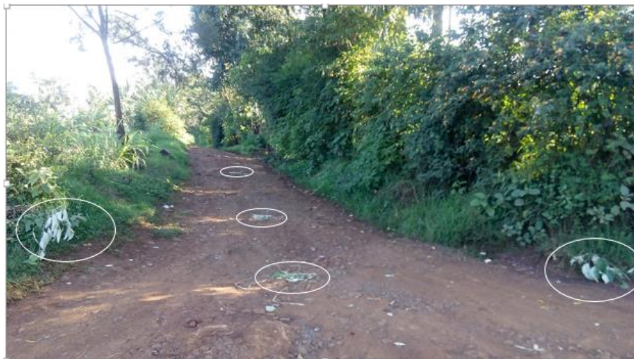
Figure 7: Twigs placed on the access road to direct veterinary doctors
