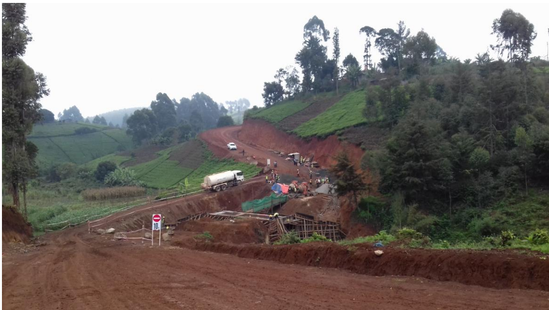
Figure 2: Construction of a bridge in Lari Sub-County
